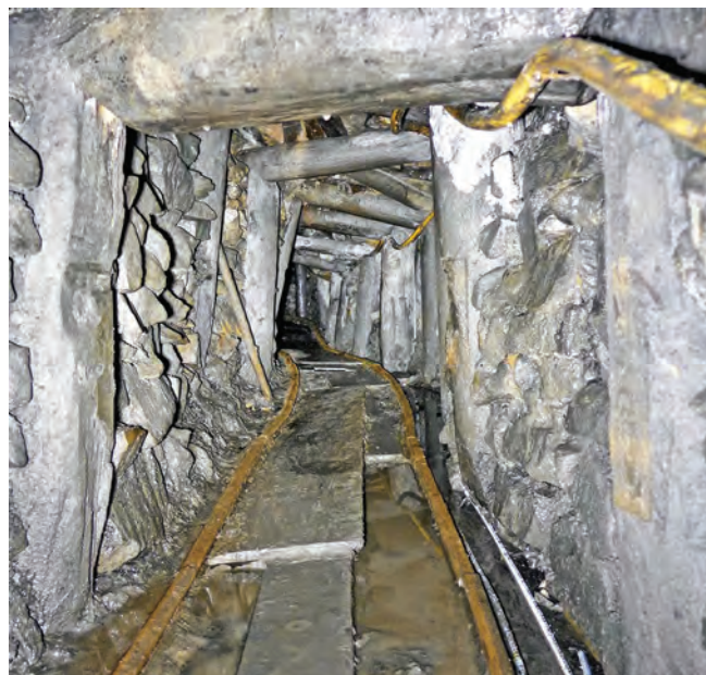
Wallsend Drift: the new haulage adit to the working face
